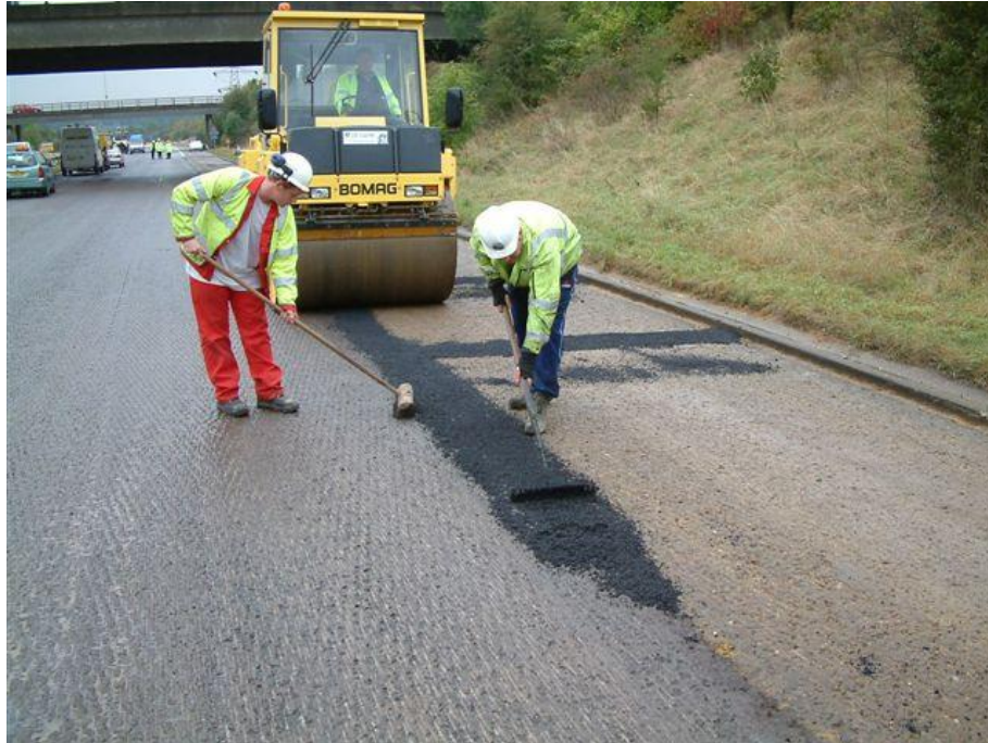
Filling excessive voids after planing the surface
