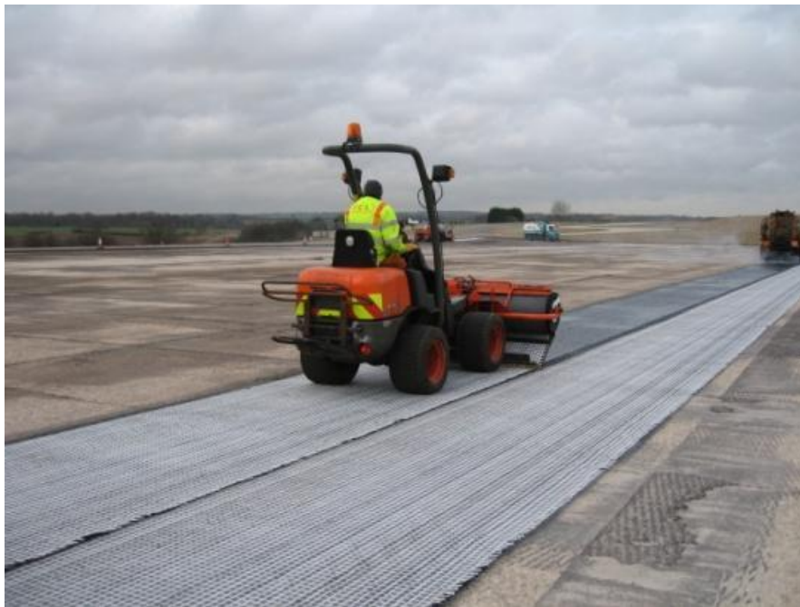
Installing a Glass Fibre Combination Grid
