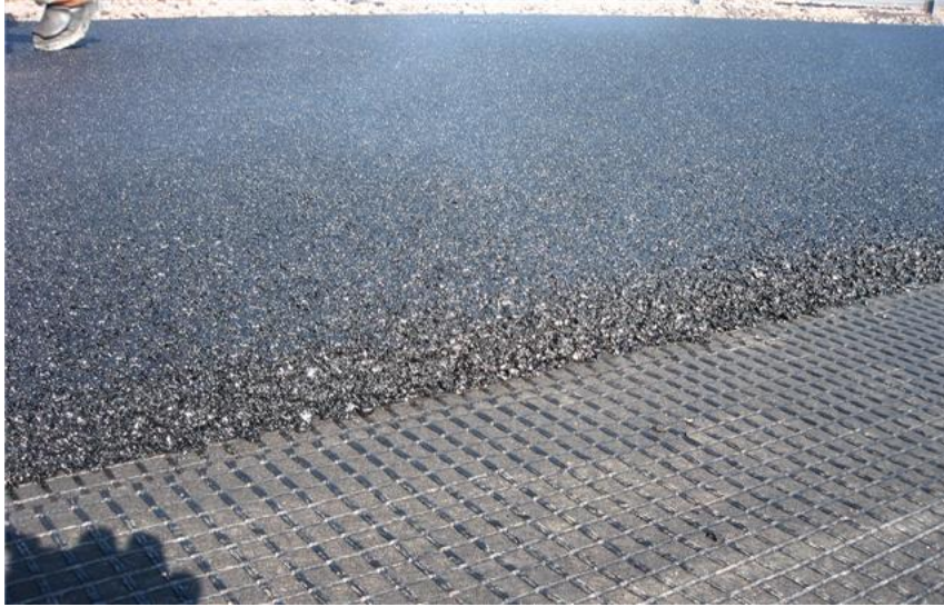
Combination Grid with Asphalt Overlay
