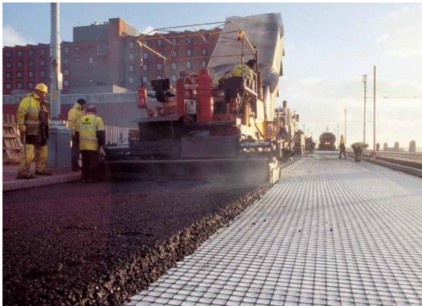
Polypropylene Grid with Asphalt Overlay
