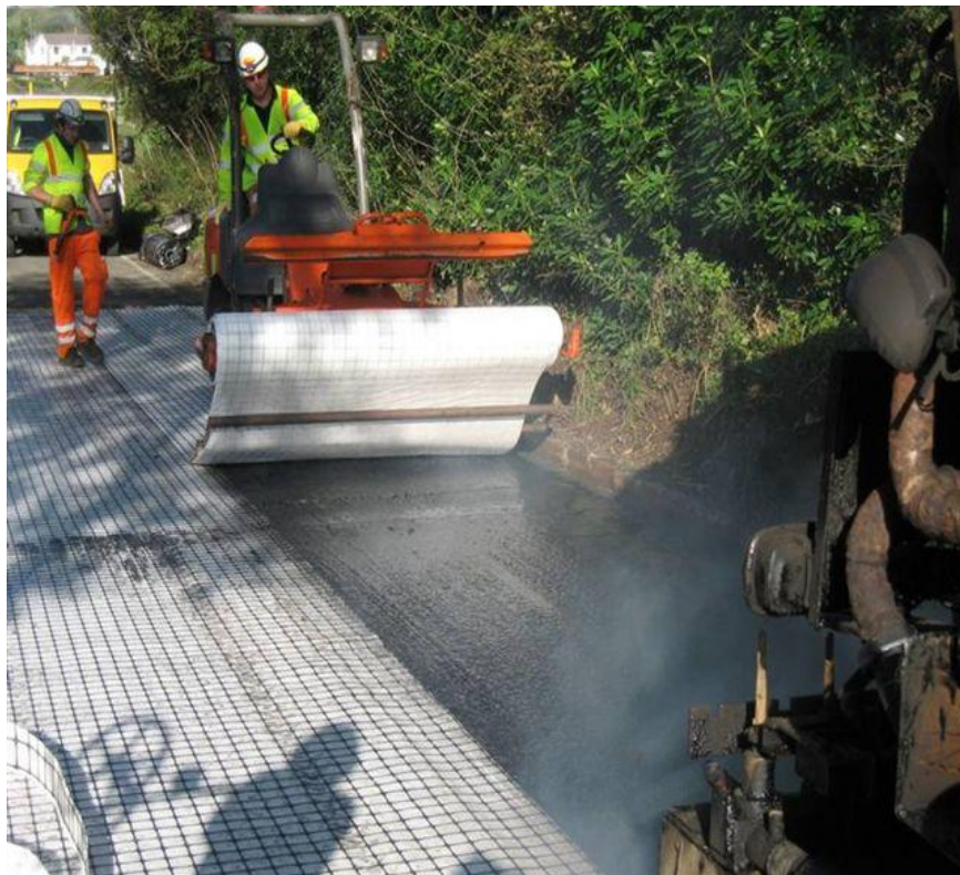
Installation of a Polypropylene Grid
