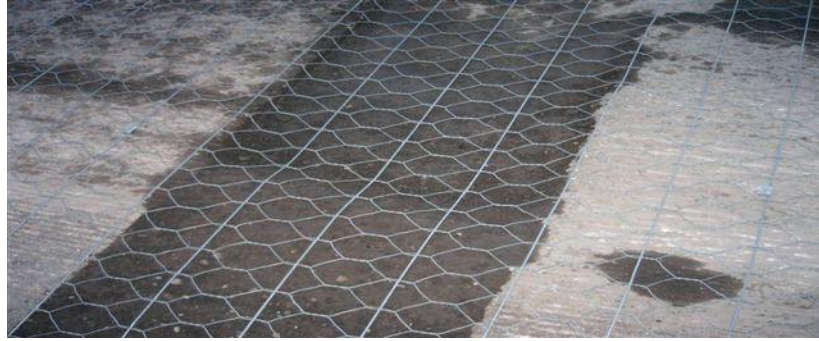
Steel Mesh Installation
