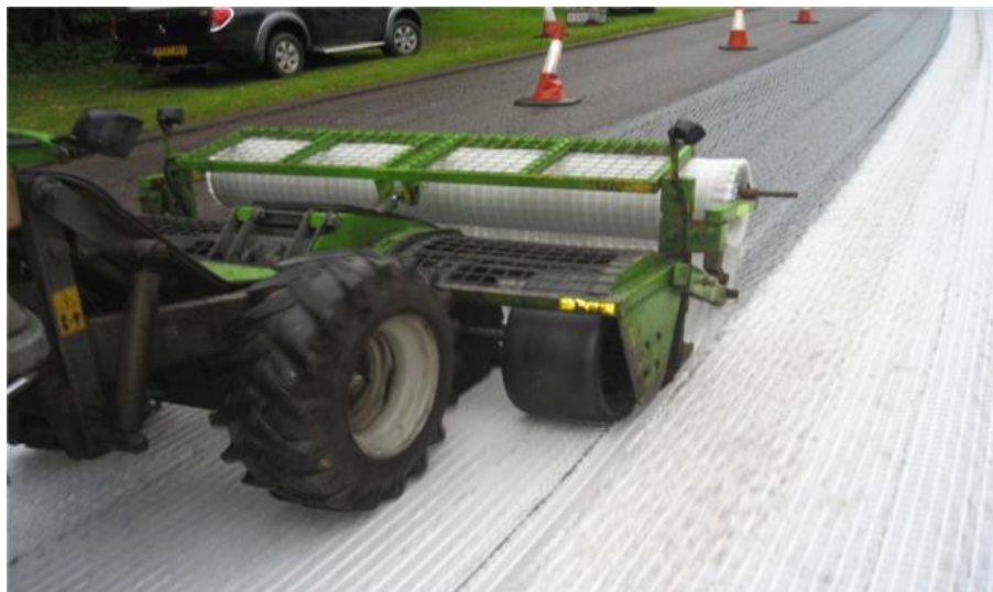
Purpose built Applicator for installing Geosynthetics
