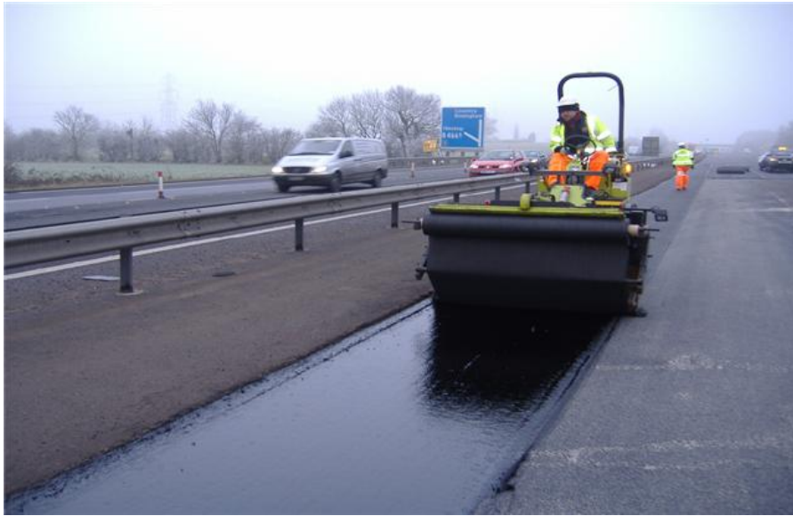
Installing a Combination Grid onto Bond Coat
