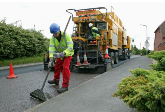
Machine applied Microsurfacing
