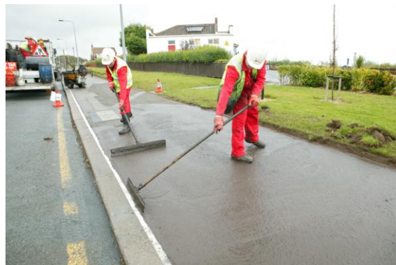
Hand applied Slurry surfacing
